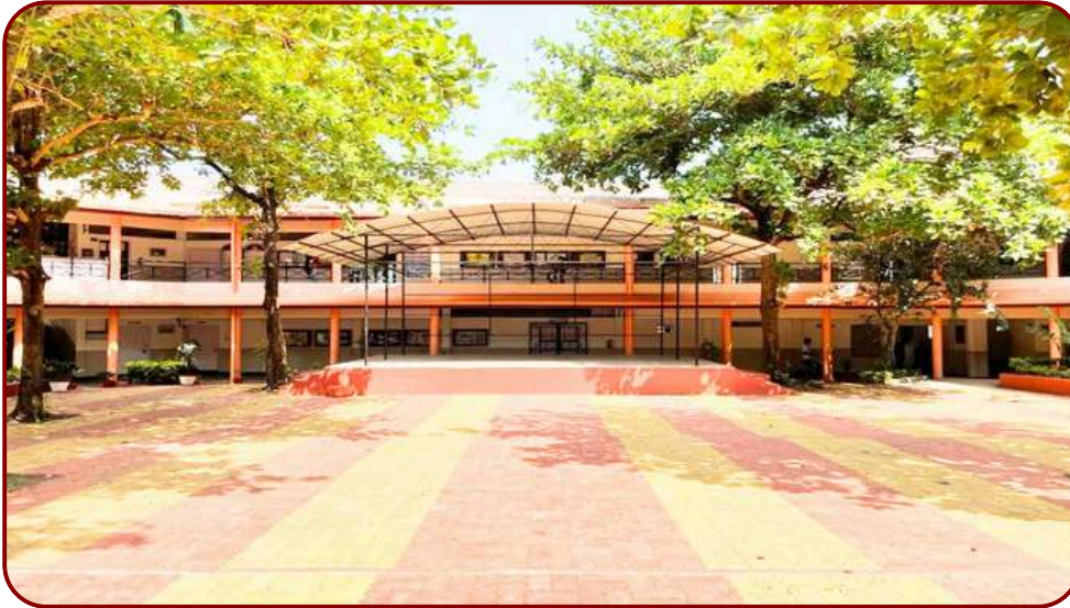
Open Air Auditorium-The Sky's the limit
