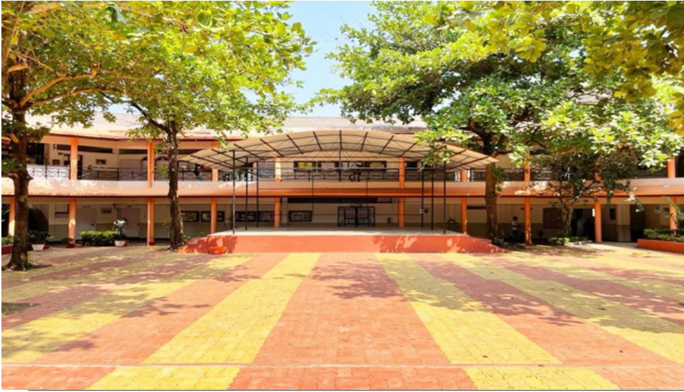
Open Air Auditorium-The Sky's the limit
